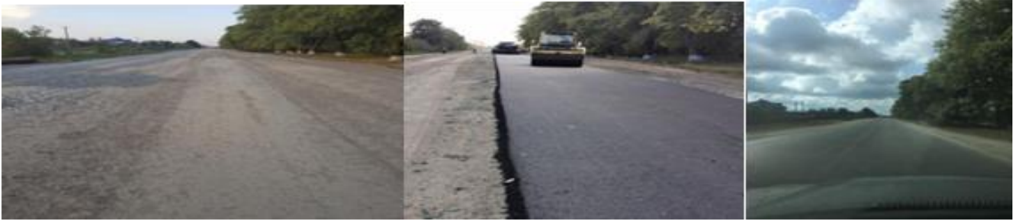
Pilot project federal road
