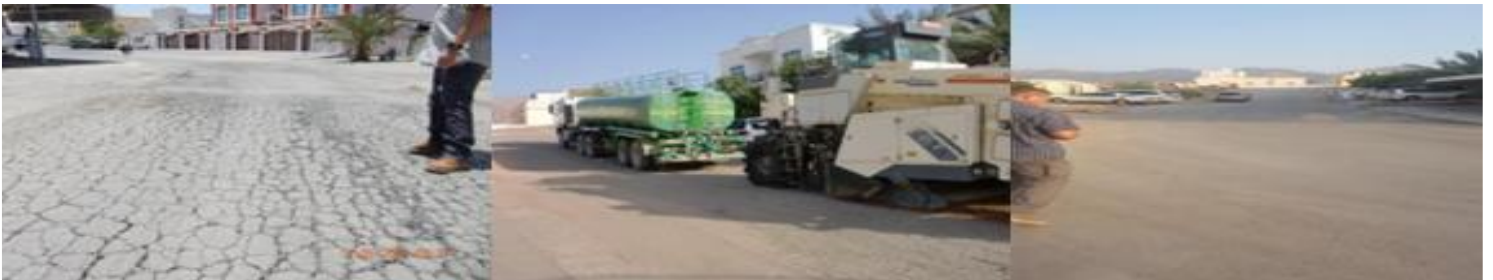
rehabilitation of Residential Area in Muskat
