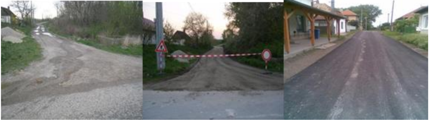
rehabilitation of local roads in 94621 Velke-Kosihv
