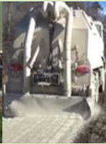
Cement spreader with Suction device
